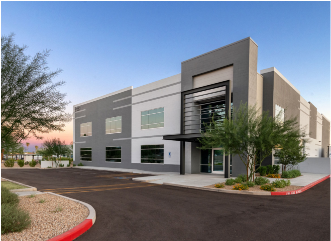
Light industrial uses
