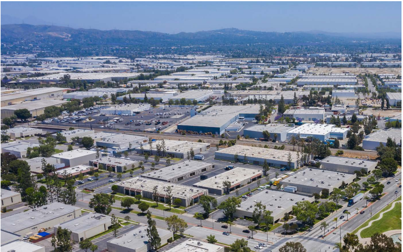
Industrial and manufacturing uses make up over 70 percent of all uses in Santa Fe Springs.
