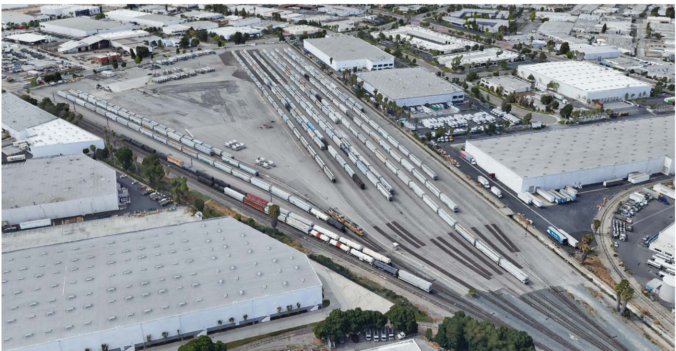
The Union Pacific Distribution Services Valla railport is a dedicated facility for plastics and some dry bulk commodities. The railyard has capacity for 250 rail car spots and is located at 8636 Sorenson Avenue.
