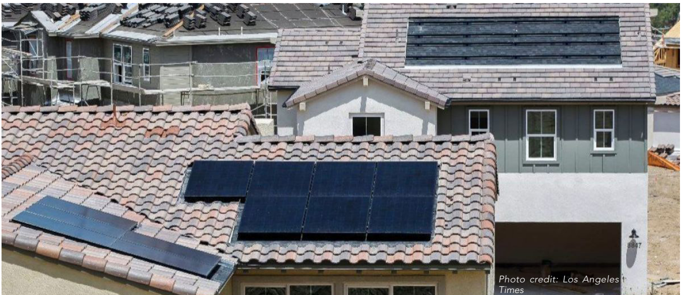
Solar rooftops on new homes under construction
