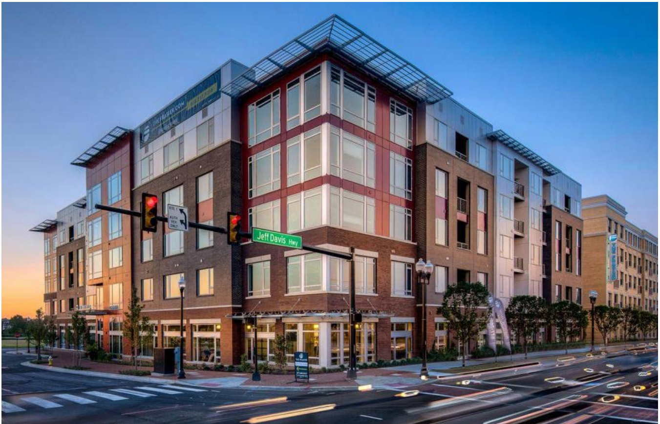
Multi-family residential uses are envisioned adjacent to the Norwalk/Santa Fe Springs Transportation Center
