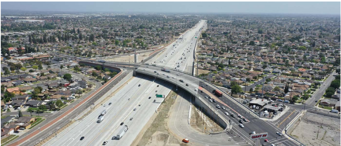
Aerial view of Florence Avenue and I-5 Freeway interchange.
