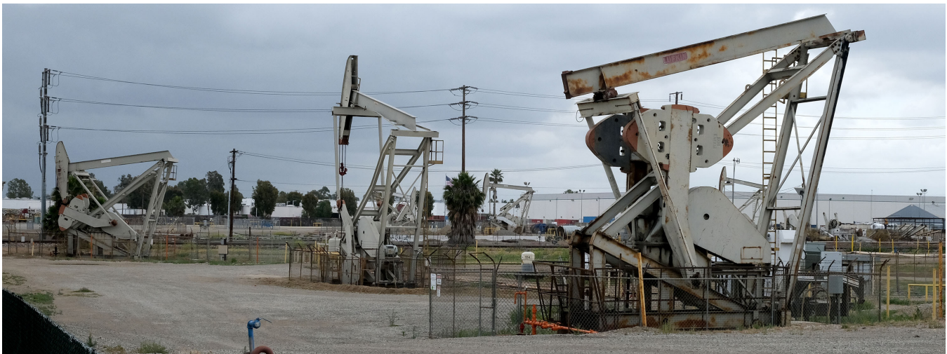
There are nearly 200 active oil wells in the community with some in residential areas.
