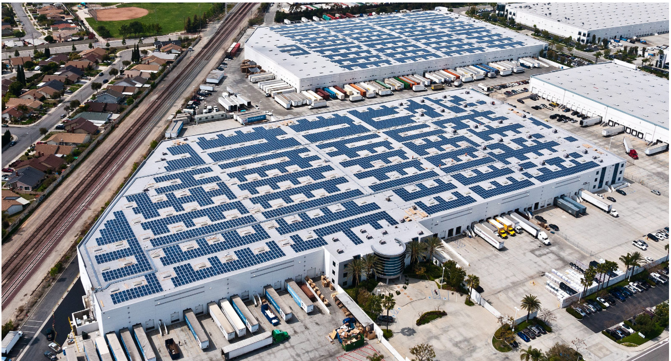
Solar panels on large industrial roof tops at the Golden Springs Business Center, are creating electricity and reducing carbon emissions, specifically carbon dioxide. Carbon dioxide, which is a greenhouse gas, is contributing to global warming and climate change.
