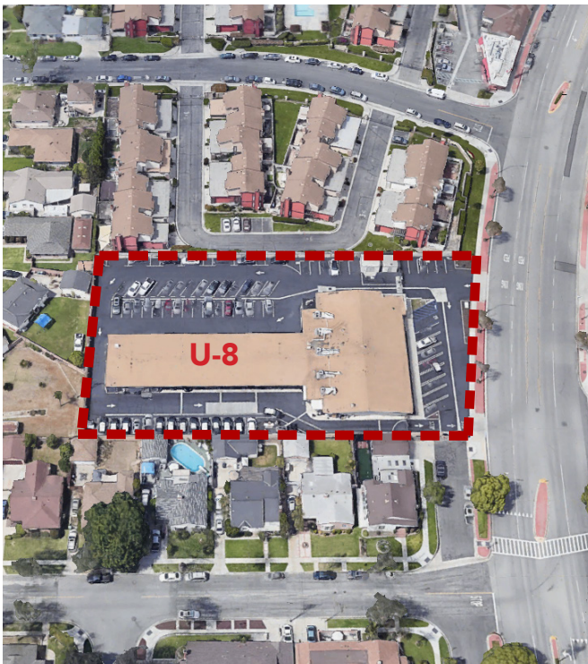
Site U-8: California Highway Patrol Site
