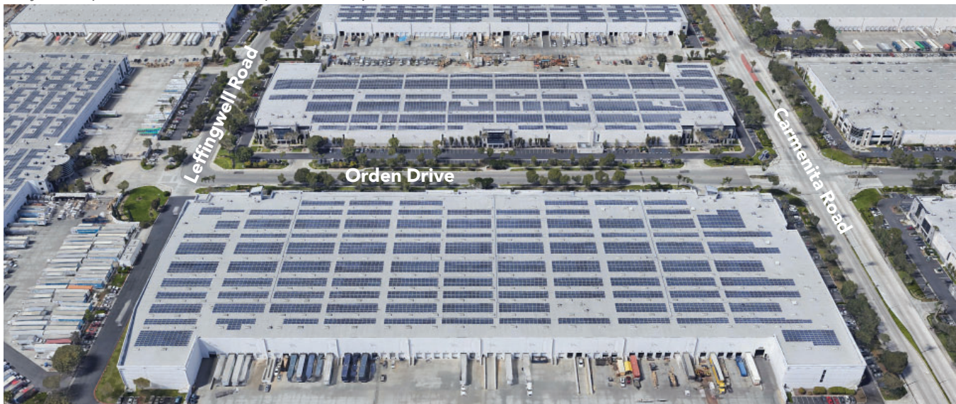
Many of the buildings in the Golden Springs Business Park include rooftop solar panels
