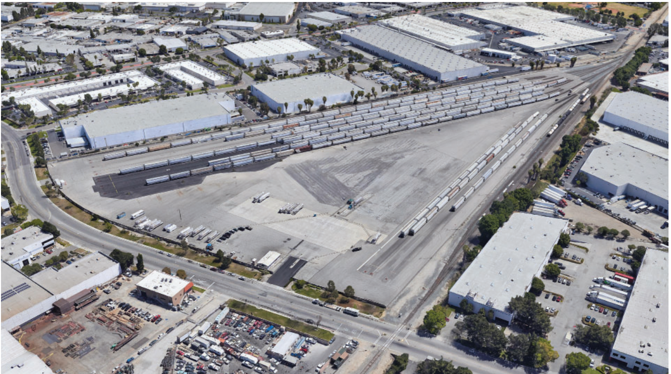
The Union Pacific Distribution Services (UPDS) Valla railport is a dedicated facility for plastics and some dry bulk commodities. The railport consists of 250 rail car spots.
