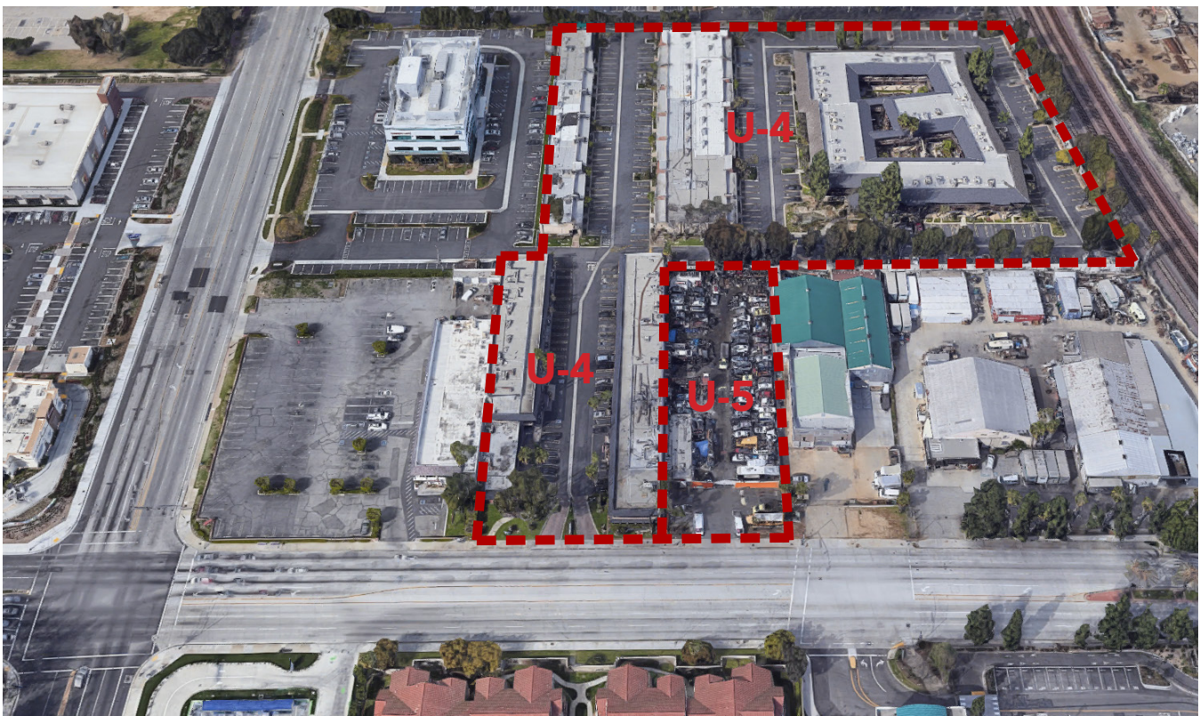
Sites U-4 and U-5: Sites near the Norwalk and Santa Fe Springs Transportation Center, with train and bus transit accessibility.
